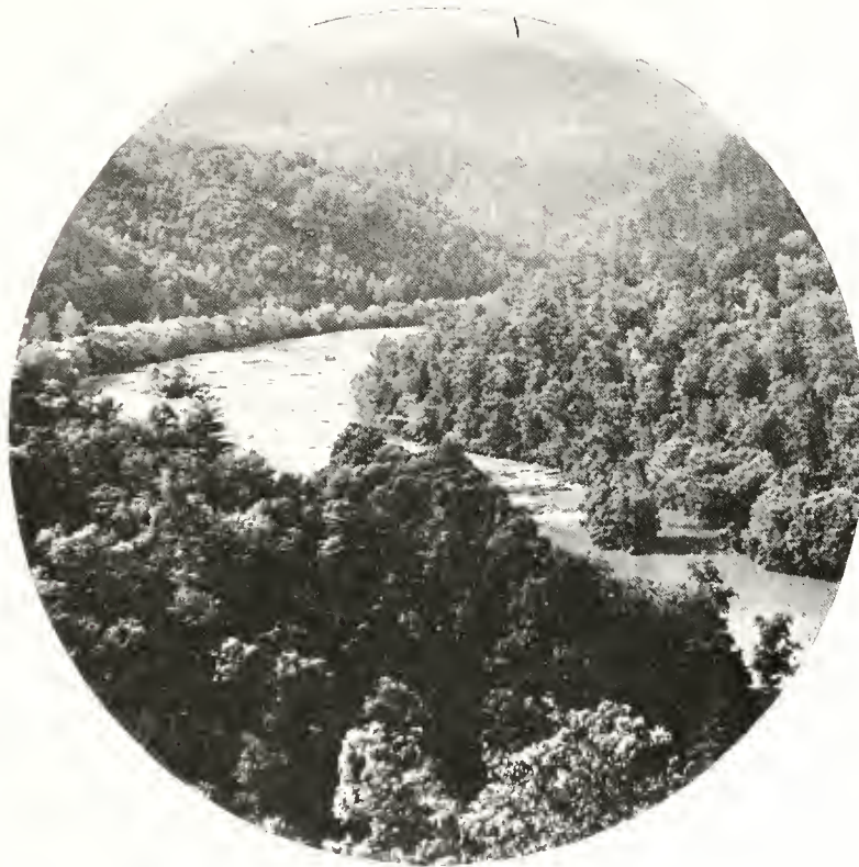
Fowler Bend, first "TVA" dam to come to North Carolina will rise between these wooded cliffs on the Hiwassee below Murphy. A temporary access road has just been constructed on the north bank, and foundations for a construction bridge are now being laid.
