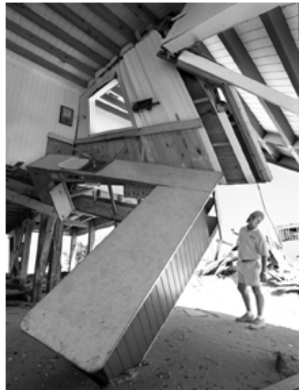
This Oak Island home was partially lifted off its foundation and grotesquely twisted.
