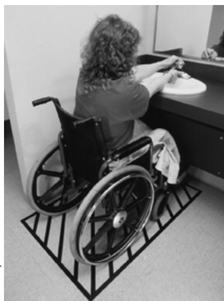
Modifying an employees’ restroom is often necessary to accommodate a person in a wheelchair, whose needs include more space to maneuver and lowered sinks with knee space below.
