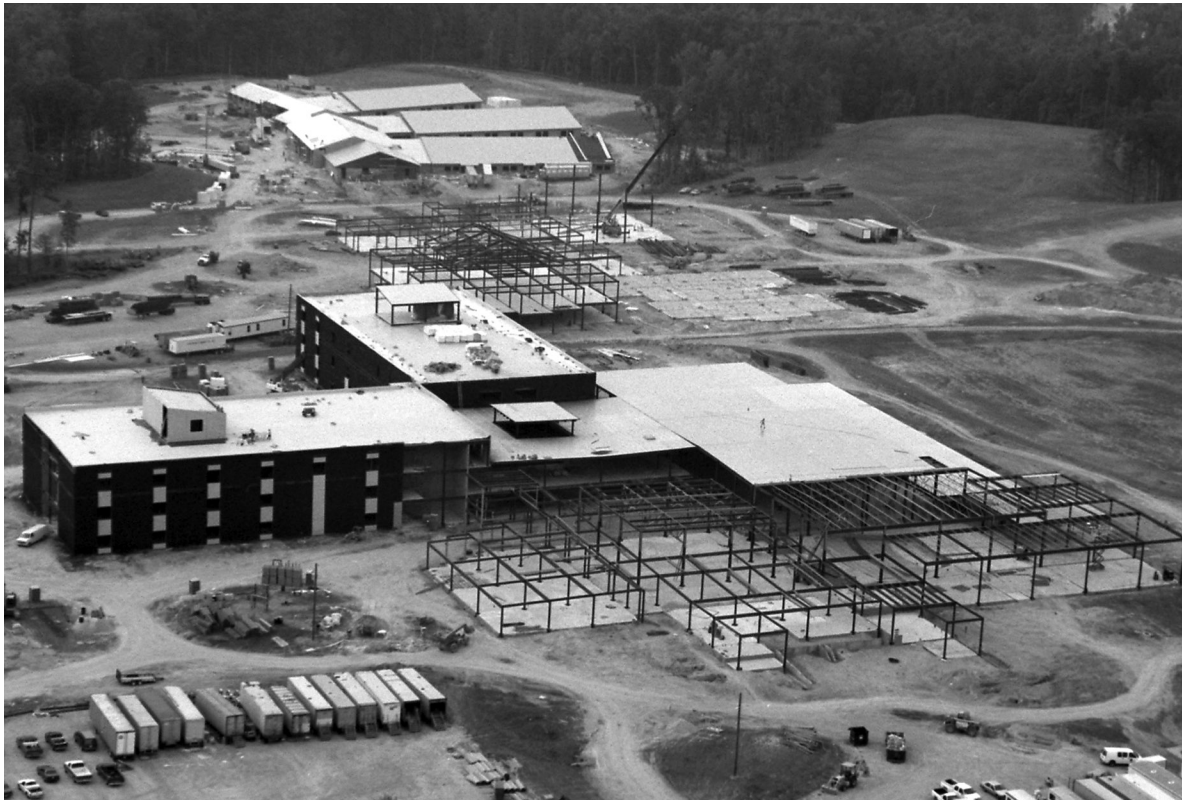
One of the new schools under construction in Wake County
