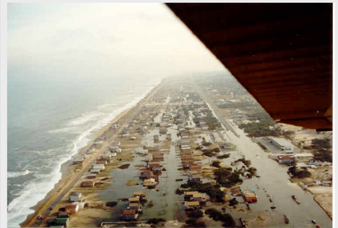
Flooding at Kill Devil Hills following Hurricane Irene. (Photo Credit: Town of Kill Devil Hills)
