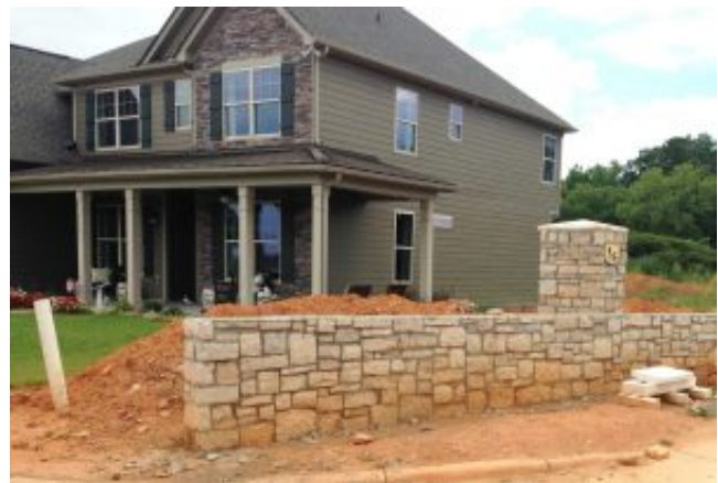
House under construction, Gastonia, N.C.
