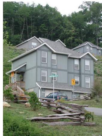
White Laurel development in Boone. 42 units of income-restricted rental housing developed in late 1990s by Northwestern Regional Housing Authority and other partners.
