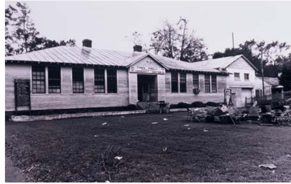
Figure 2: Princeville Town Hall, showing the water level of the flood from Hurricane Floyd, 1999
