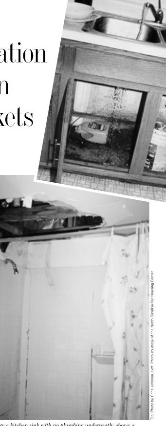
Top: a kitchen sink with no plumbing underneath; above: a gaping hole in the ceiling over a shower.
