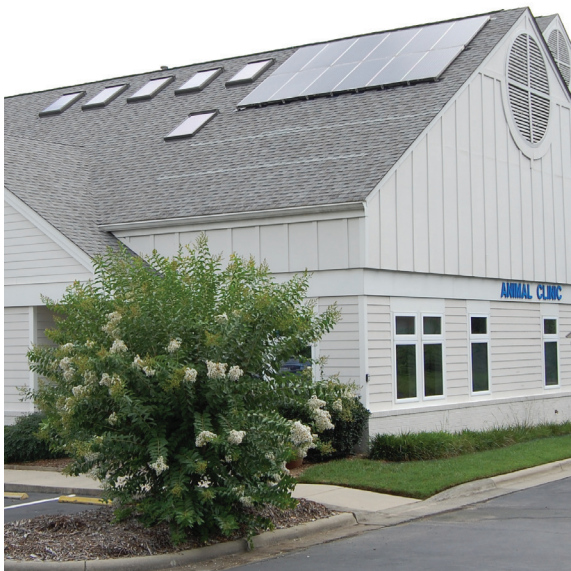
Flush-mounted solar panels on a pitched roof.
