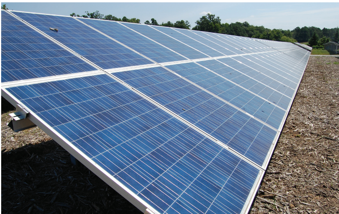
Photovoltaic panels (or modules), here on a solar farm, convert sunlight into electricity.
