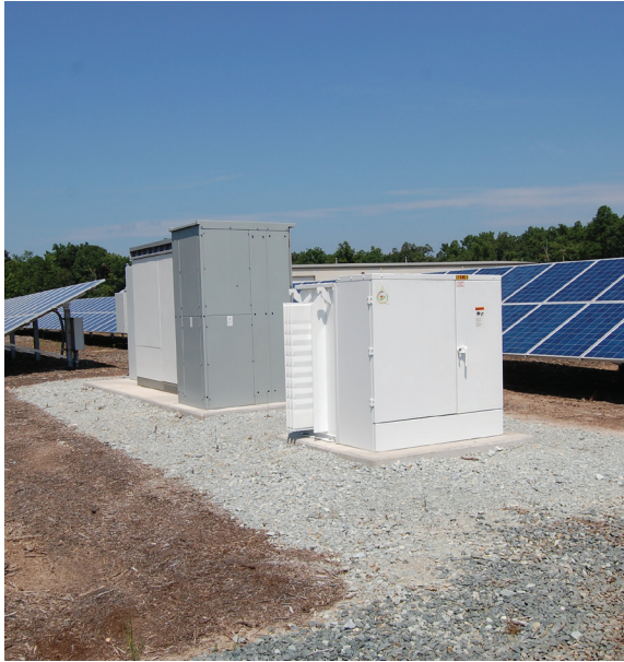
Inverters—the equipment needed to convert the current from DC to AC—create a minor amount of noise.
