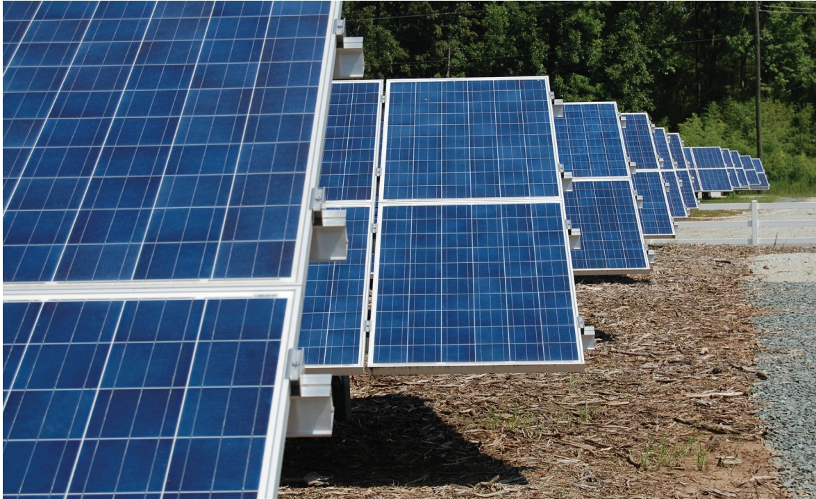
Solar cells are combined into solar panels, solar panels are combined into solar arrays, and solar arrays are combined into a solar farm, such as in this solar farm in Chatham County.
