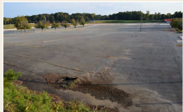
The footprint of the old Eastland Mall remains as efforts for redevelopment continue.
